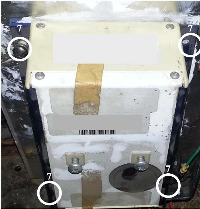
7. Remove the 4 Phillips head screws securing the control to the panel and remove the control.
